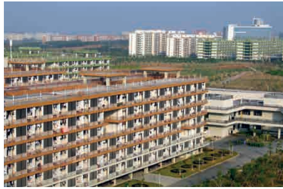
Figure 5.5-5 Large-scale residential projects in Guangzhou. Source: Frauke Kraas/WBGU
