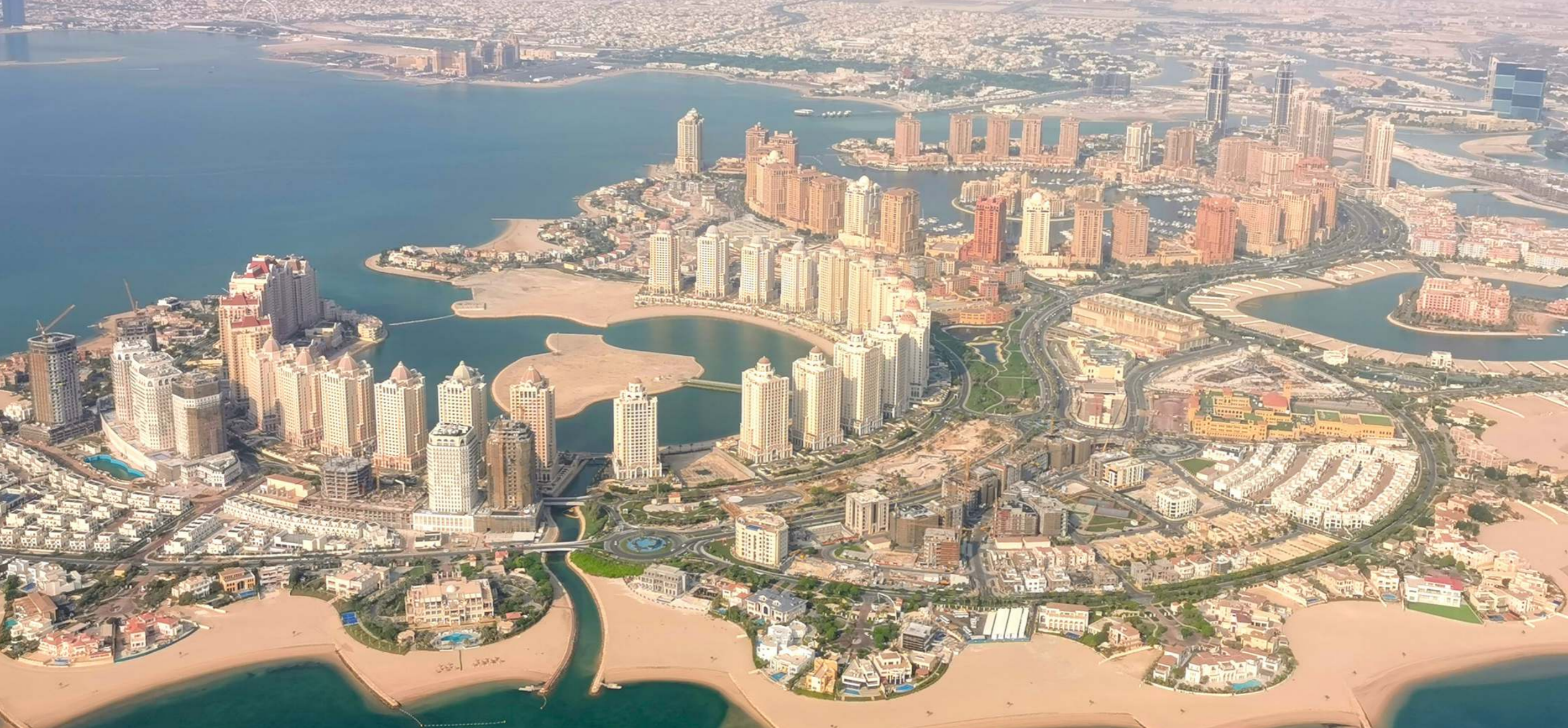
Image Source: The polder area of "The Pearl" in Doha, Qatar, with Bariya Beach (foreground) and Marsa Arabia (background) Marina. A real estate and infrastructure project worth over $10 billion led by UDC-United Development Company, a Qatari investment company. The Pearl is located on over 4 million m 2 of reclaimed land. September 2022. Image by Nicolas J.A. Buchoud, all rights reserved ©.
