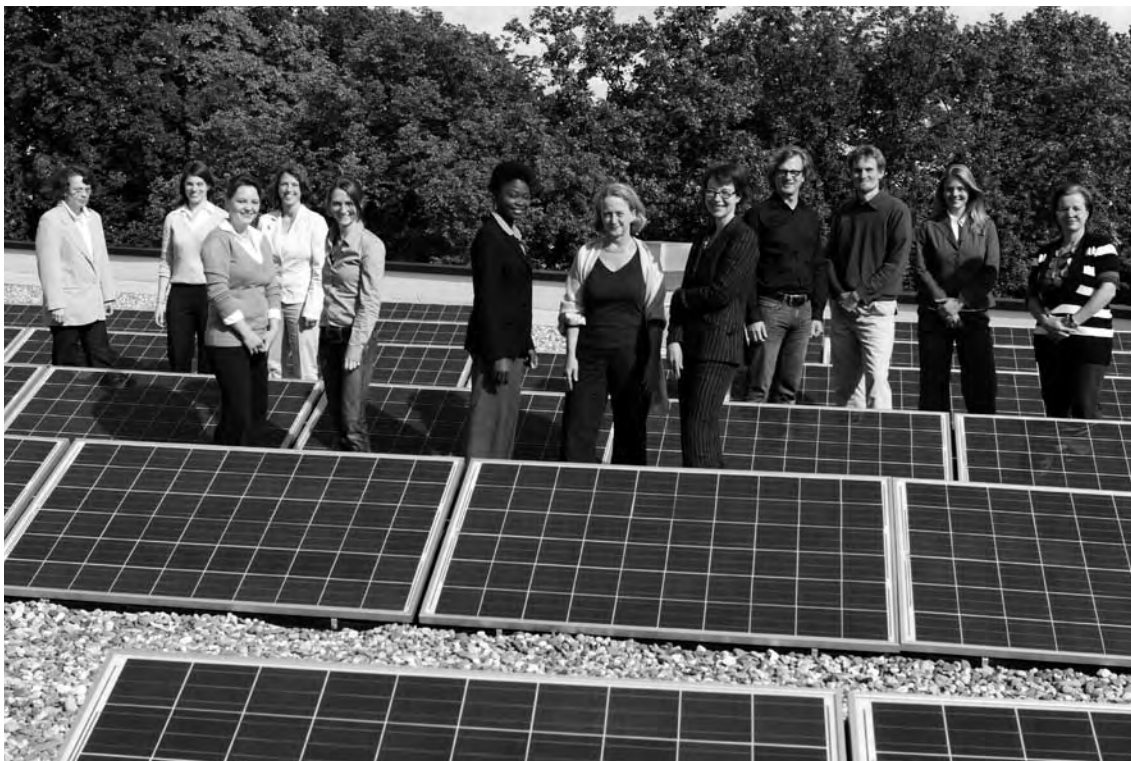
Solarworld Photovoltaic elements, Building PO 1, Bonn
